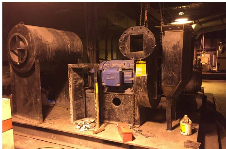
Flotation Blower #3 Installation
